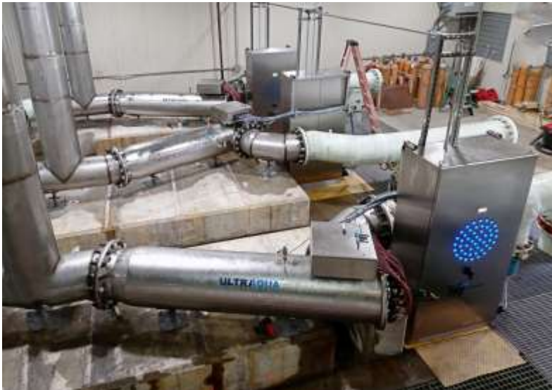
3x MR48-350SS, each treating 1500 m 3 /h Ed Weed – Grand Isle in Vermont, USA
