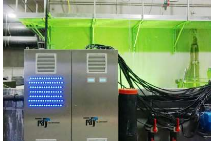
2 x MR100-350SS Channel, each treating 2600 m 3 /h in AquaPri, Denmark
